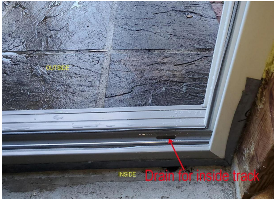
Figure 1: Drain holes on the interior track
