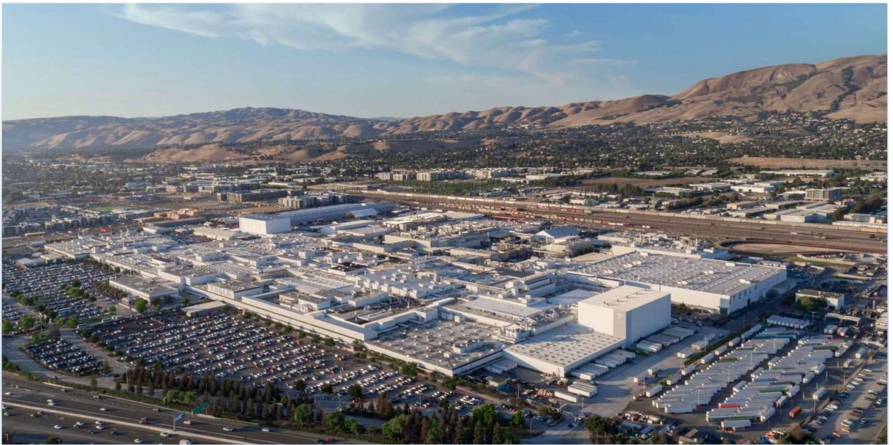
24 Tesla's 5.3 million square foot factory in Fremont, California.
