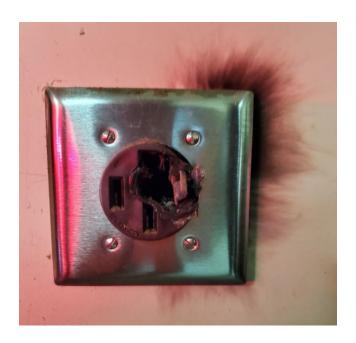
33. Similarly, on or about January 3, 2023, another Taycan owner found that the included supply cable, plugged into a NEMA 14-50 outlet, had melted both the outlet and the cable's plug:28
