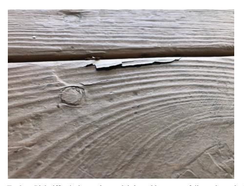
91. To date, Plaintiff's deck remains unsightly and in a state of disrepair, as the RockSolid 2X still cracks, chips, strips, and otherwise fails and degrades.
