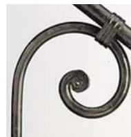
Hand-forged iron scrollwork and joinery.
